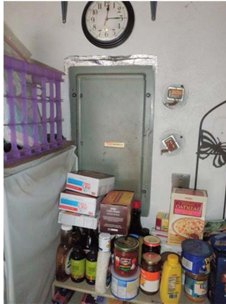
Electrical Panel Photo
